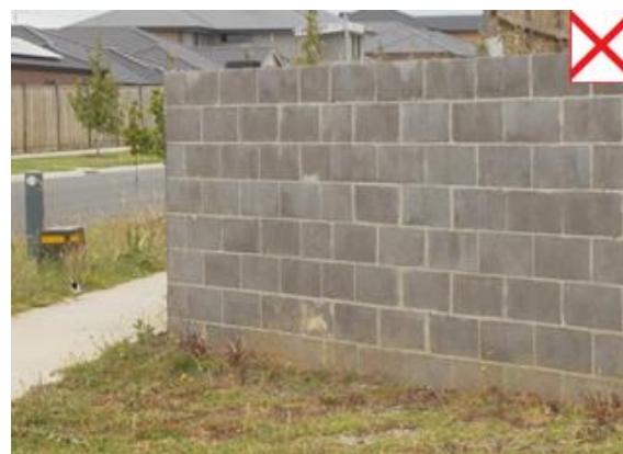
Unfinished Concrete Retaining Wall
