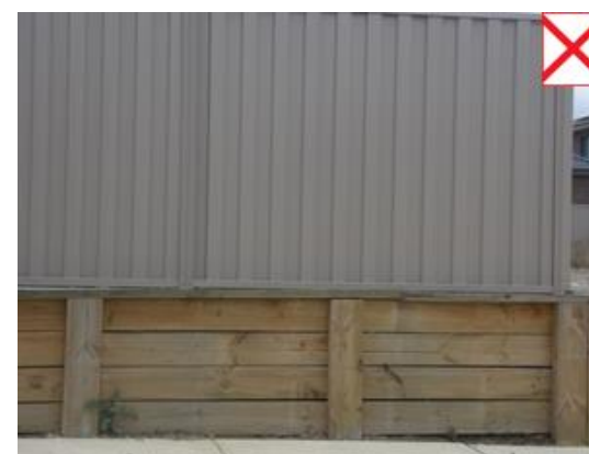
Unfinished Timber Retaining Wall
